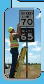
When signs are installed, the installation date is labeled or recorded. The age of the sign is compared to the expected sign life. Signs older than the expected life should be replaced.
